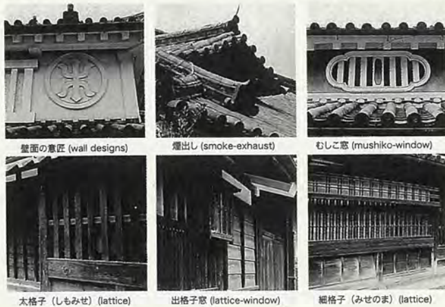
壁面の意匠 (wall designs) 煙出し (smoke-exhaust) むしこ窓 (mushiko-window) 太格子 (しもみせ) (lattice) 出格子窓 (lattice-window) 細格子 (みせのま) (lattice)
